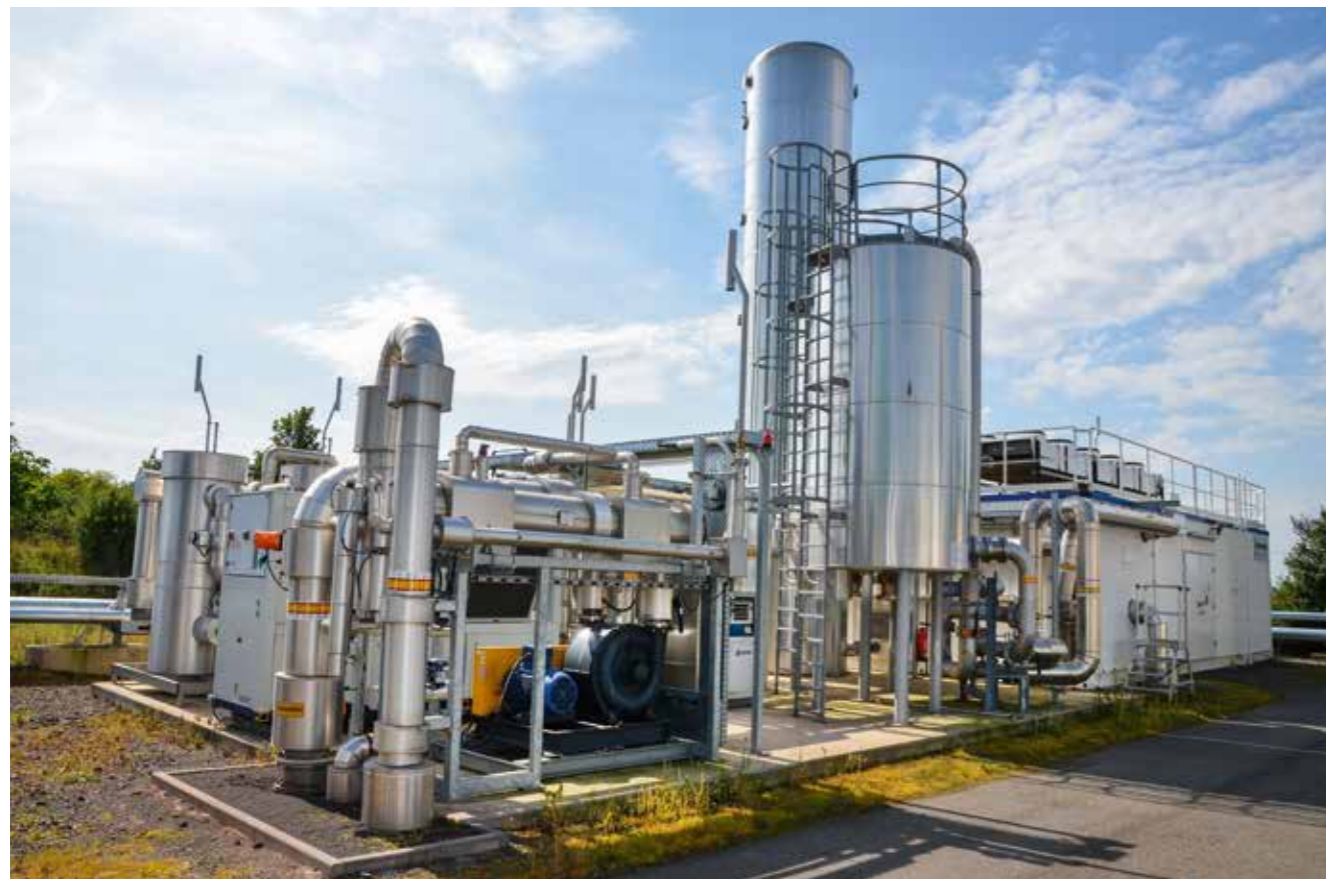
Gas treatment is based on pressure-less amine scrubbing.
