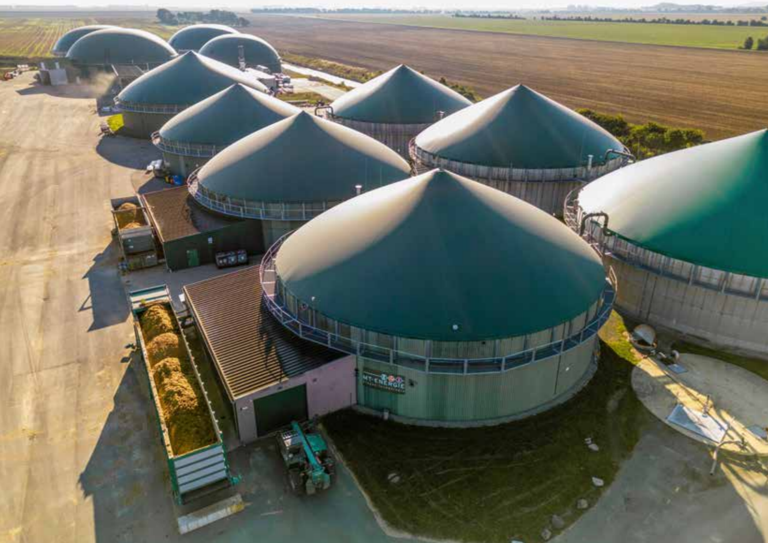
The GraNottGas digester produces 4.5MW of electricity. It is operated on a wide range of different substrates including straw, farmyard manure, dried poultry manure and slurry.
